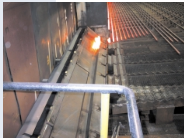
Figure 2. Tube transfer station at Vallourec & Mannesmann, Mülheim, Germany
